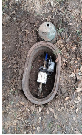
Meter Endpoint Installation- Package I & II
