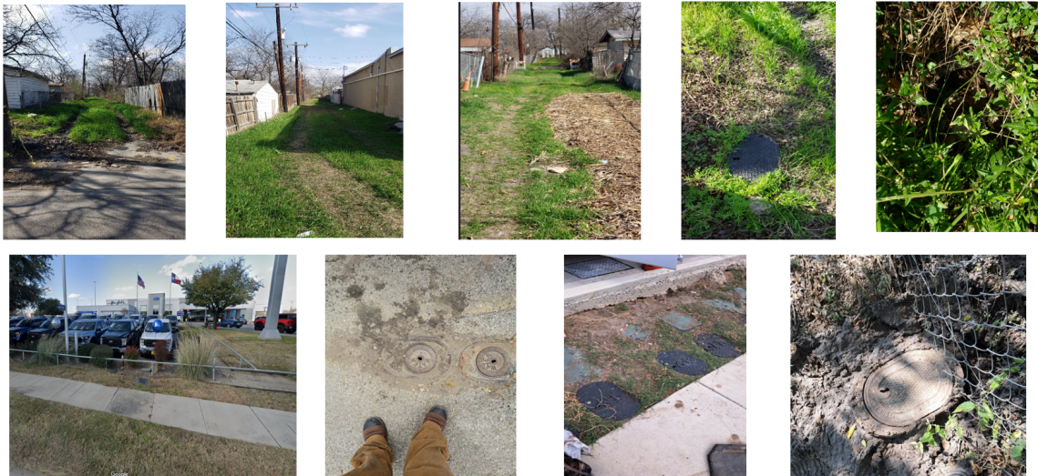
Meter Endpoint Installation- Package I & II
