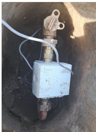
Meter Endpoint Installation- Package I & II
