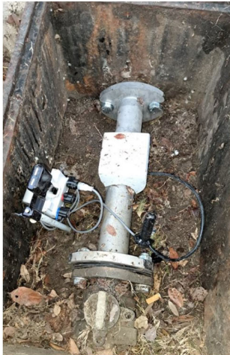
Meter Endpoint Installation- Package I & II
