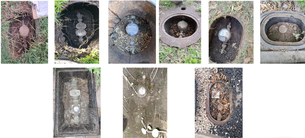
Meter Endpoint Installation- Package I & II
