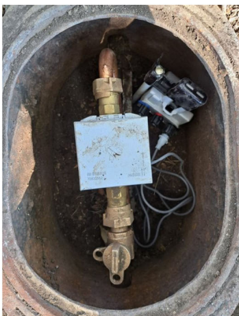
Meter Endpoint Installation- Package I & II
